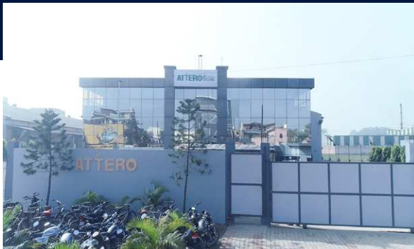
ATTERO RECYCLING FACILITY
