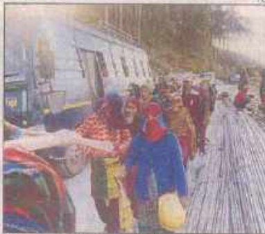
The women workers, clad in woollens and armed with shovels and construction tools, at the tunnel site on Sunday
