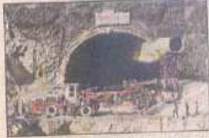
Five-member panel will recommend safety measures to be taken up during construction within 45 days
