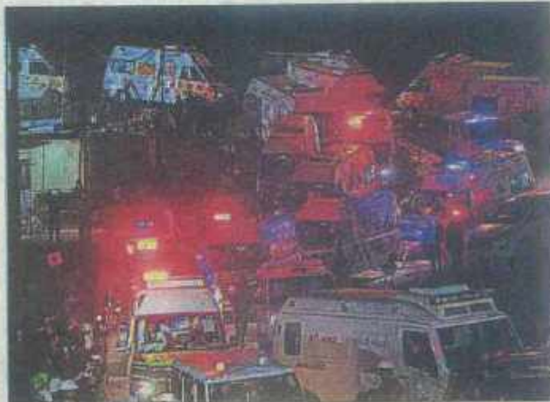
A line of ambulances carry workers rescued from the site of an under-construction road tunnel that collapsed in Uttarkashi on Tuesday. AP
