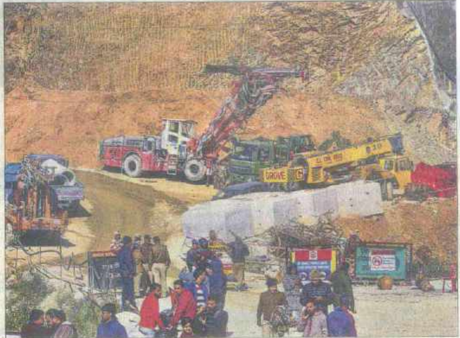
Rescue operations underway to extract 41 workers trapped inside the Silkyara tunnel.
