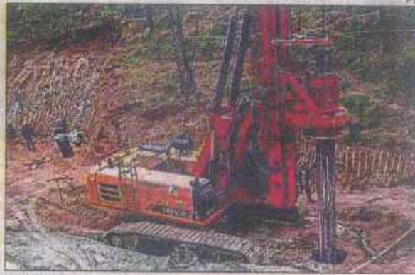
Drilling from top underway during the rescue operation on Sunday
