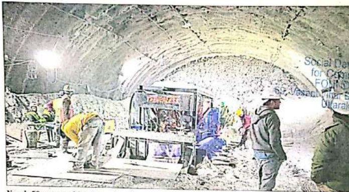
Nearly 50 metres of debris needs to be penetrated to insert the evacuation tubes.
